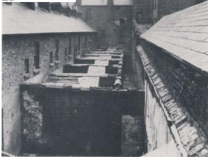
Fig. 5. Rear view of houses in Smithfield. A requirement of housing bye-law was for each house to have a yard at least ten feet square with a separate privy (dry closet). A privy roof can be seen in each yard, also the common entry at the back used for emptying refuse from the houses and conveying the contents of the earth privies and ashpits to the outside street.
